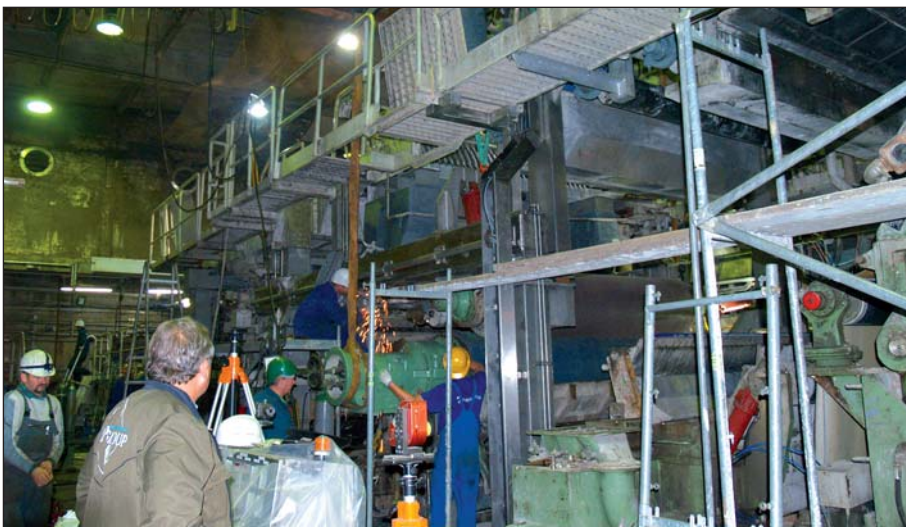
Assembly of PMP equipment at Customer's site
